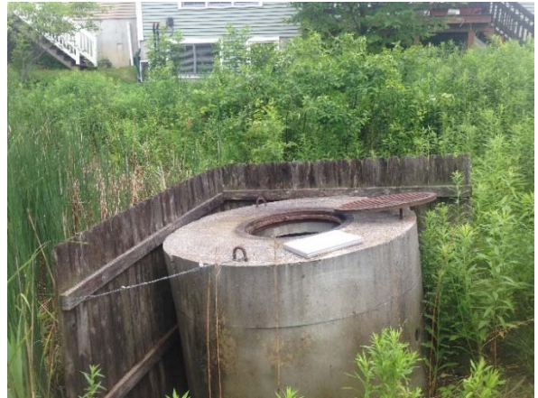
Figure 4: The Commons North Pond Outlet Structure
