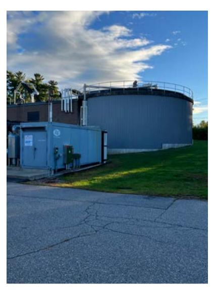
150kW co-generation system and anaerobic digester at the Waste Water Treatment Facility
