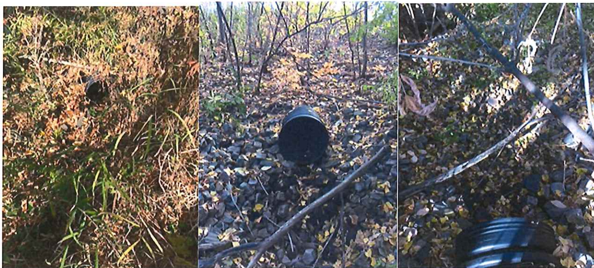
12 inch culvert proposed to be increased to 30 inch. Far left- OF 1159 inlet located in proposed gravel wetland, Center-Outfall 1160 on other side of Main Street, Right-Outfall 1160 daylight
