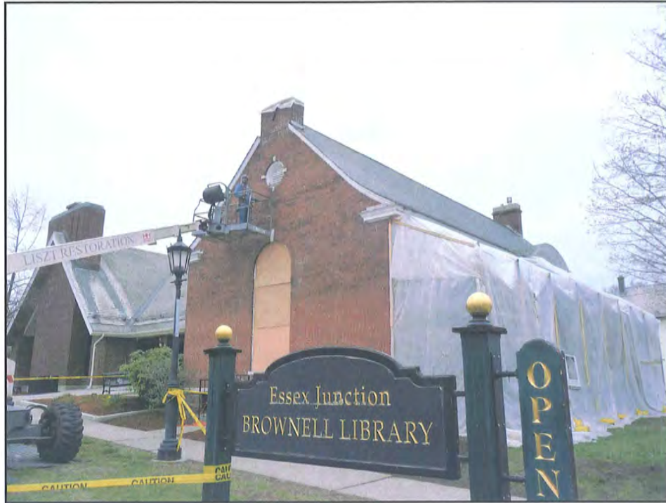
Brownell Library Exterior Rehabilitation
