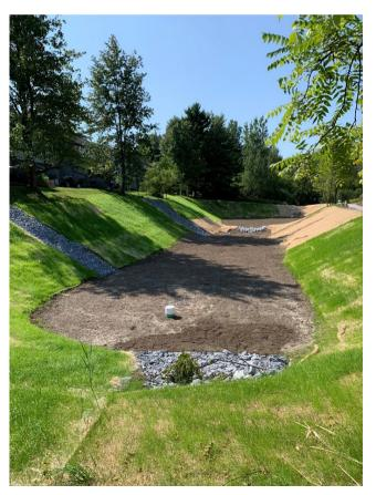
The new, completed stormwater constructed gravel wetland located at the corner of Mansfield Avenue and Brickyard Road
