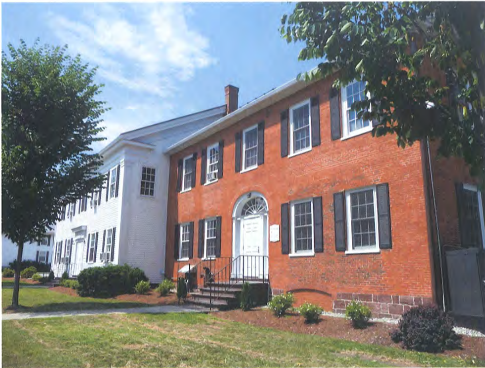
Lincoln Hall Exterior Rehabilitation Project
