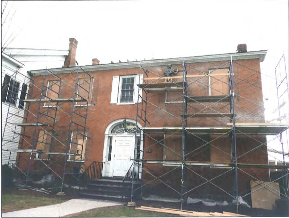
Lincoln Hall Exterior Rehabilitation Project
