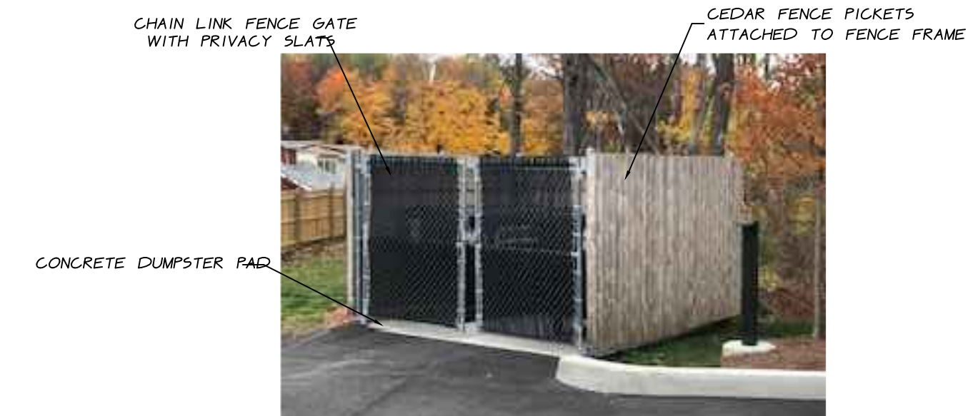
FENCE DETAIL/DUMPSTER ENCLOSURE NTS
