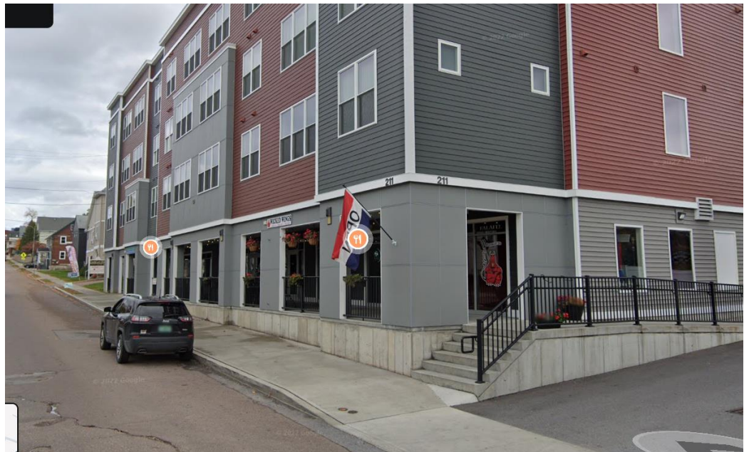
Figure 1: Example of building on a slope with terraced outdoor space in front of building at 211 Main Street, Winooski VT
