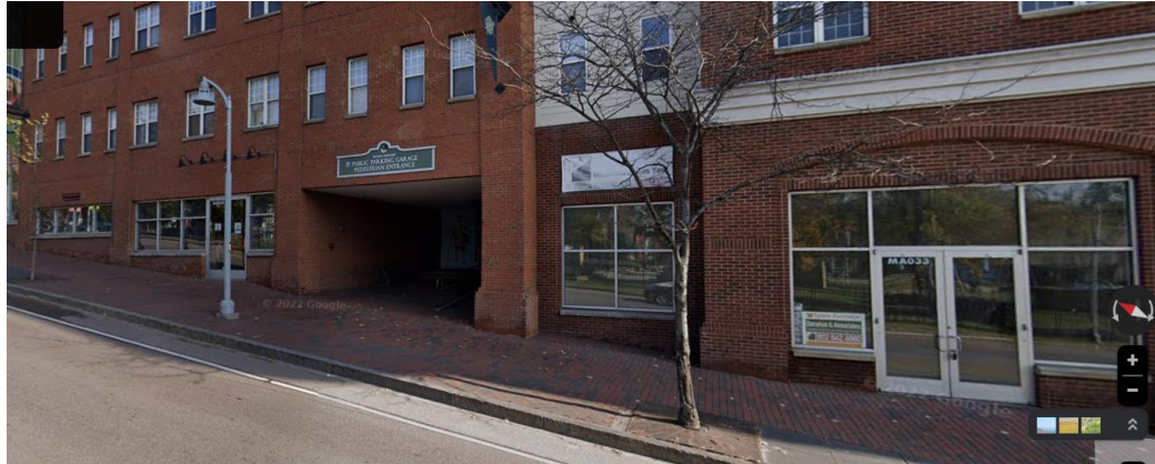
Figure 2: Example of building on a slope with an indoor layout that enables direct sidewalk access at multiple business entrances. 25 Winooski Falls Way, Winooski VT
