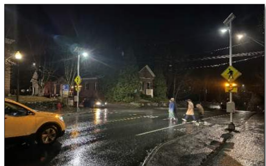
Example of RRFB with Activated Street Lighting
