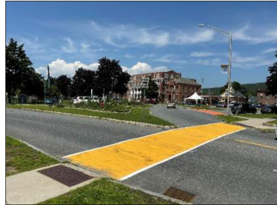
Crosswalk Painted Yellow to Improve Visibility
