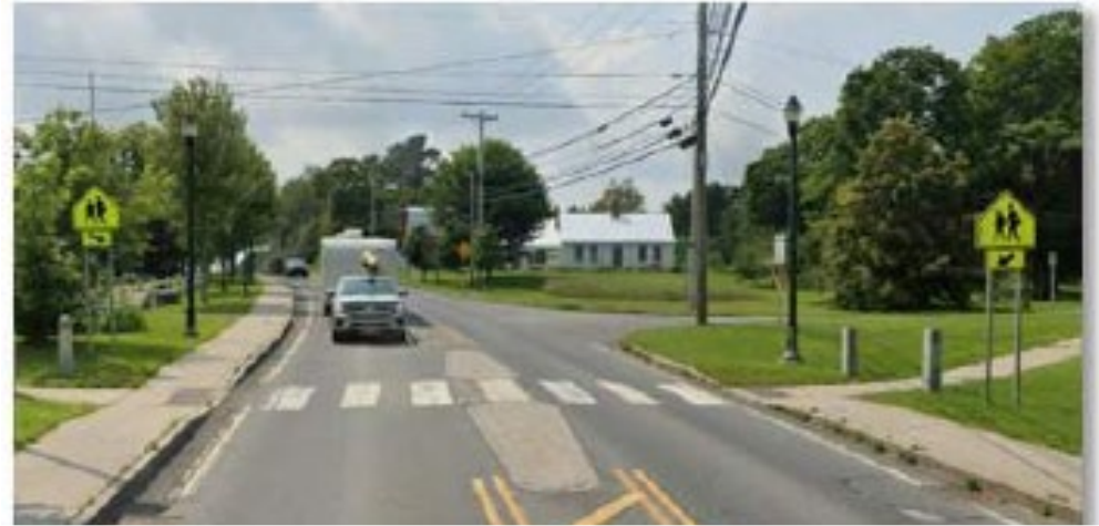
Example of a Flush median in Danville, Vermont – Stamped Concrete with Granite Edging
