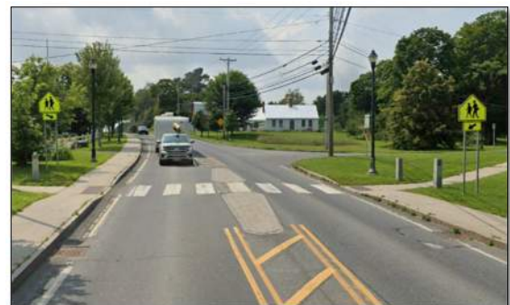
Example of a Flush median in Danville, Vermont – Stamped Concrete with Granite Edging
