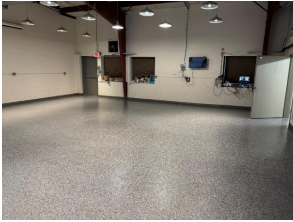
New Liquid Stone Epoxy surface on the training and fingerprint room floor.
