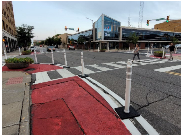
Figure 7: Temporary curb extension in South Bend, IN
