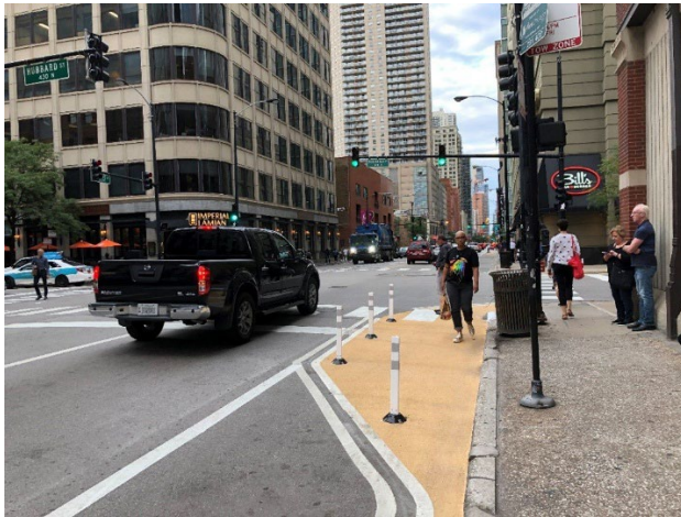
Figure 6: Temporary curb extension in Chicago, IL
