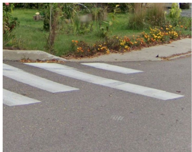
Figure 2: Street view of elongated vehicle stop bar conflicting with crosswalk striping. Source: Google
