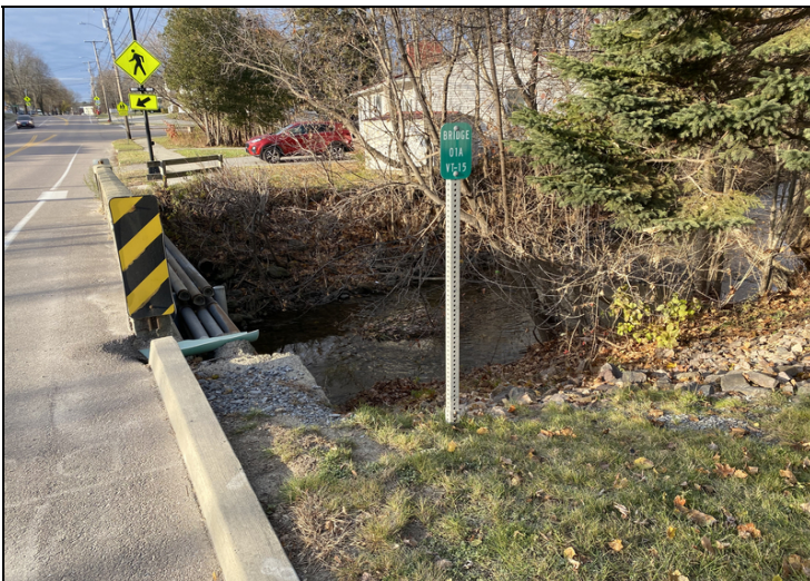
Lack of Approach Rail Downstream
