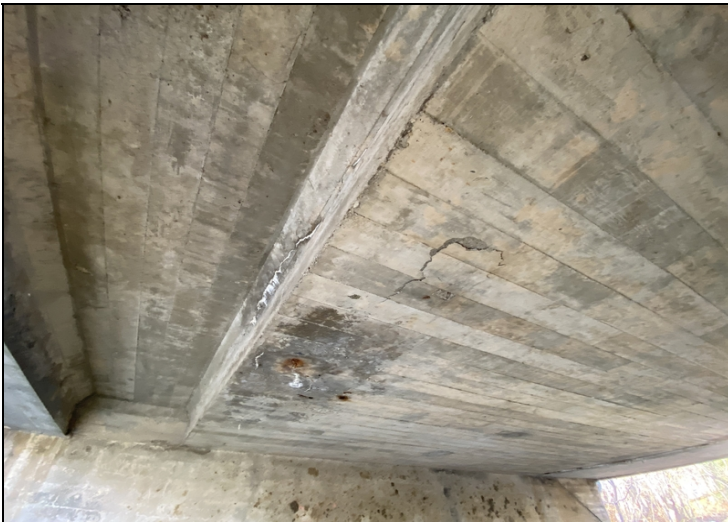
Small delam, small area of saturation and cracking with efflorescence.
