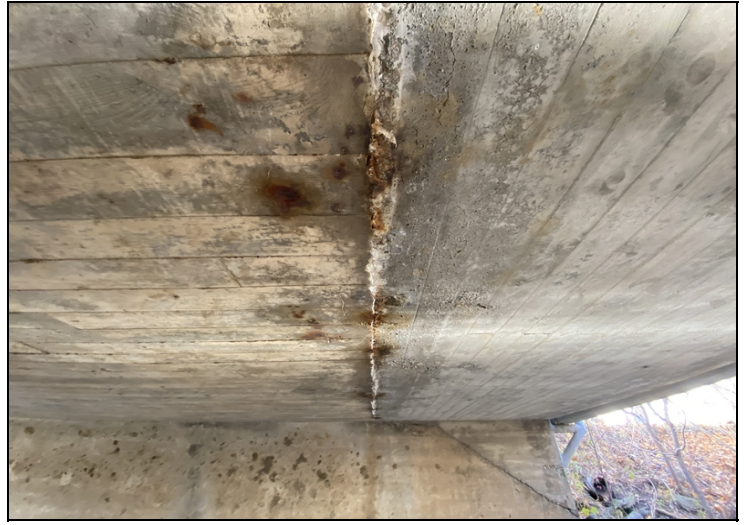
Leakage with efflorescence and rust staining at construction joint.
