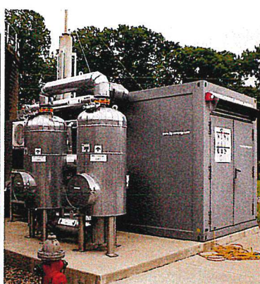
105 kW methane cogeneration installation
