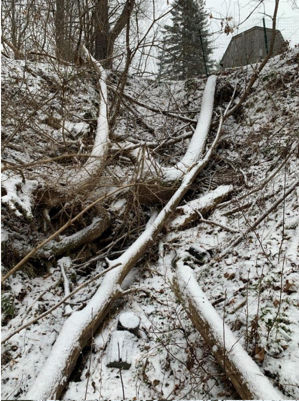
Close-up of gully erosion at outlet
