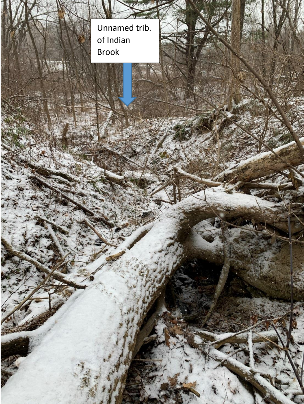
View from top of outlet 1074. This shows the gully erosion present as of Nov 2020
