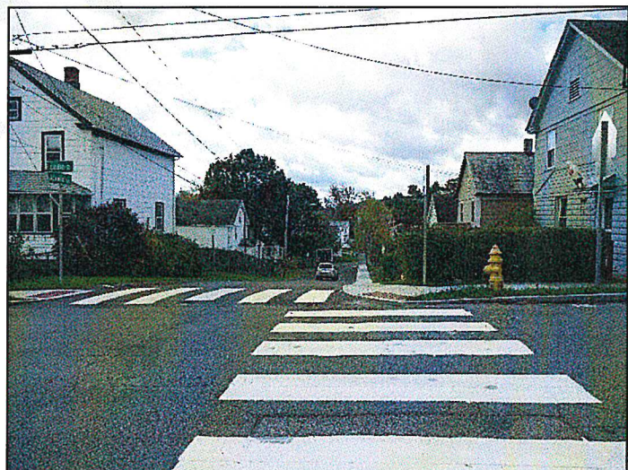
Figure 5: Example compliant ramp and crosswalk markings.
