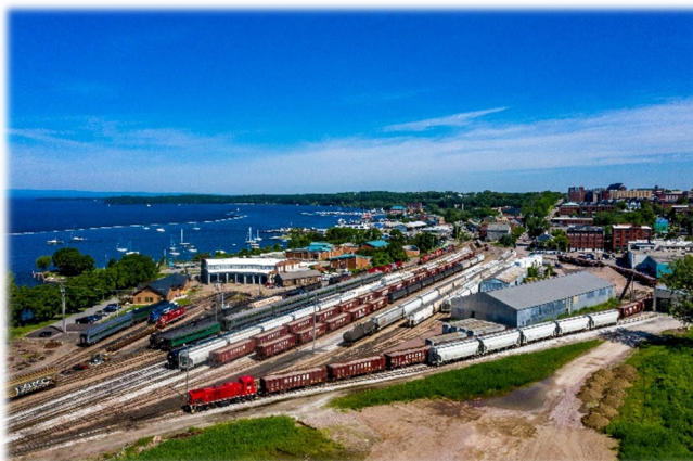
Figure 7: 2019 Aerial View of Existing Burlington, VT Railyard
