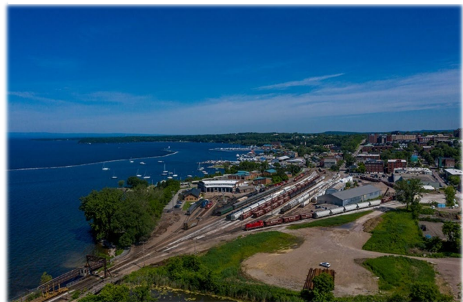
Figure 1: 2019 Aerial View of Existing Burlington, VT Railyard
