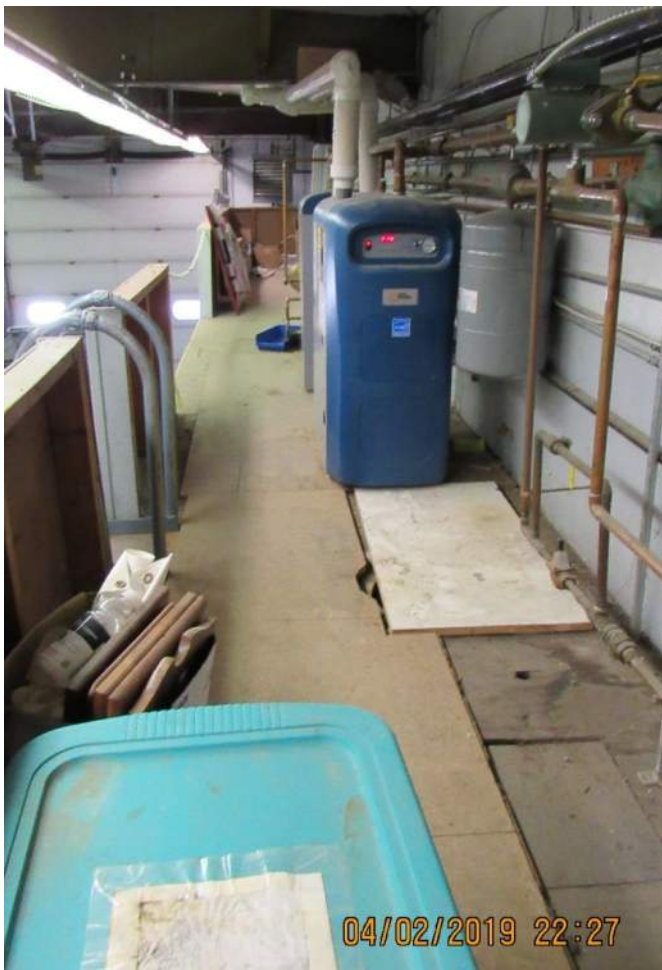
Boiler Room "Mezzanine" with Boilers; Note plastic storage boxes, damaged wood floor and walls.
