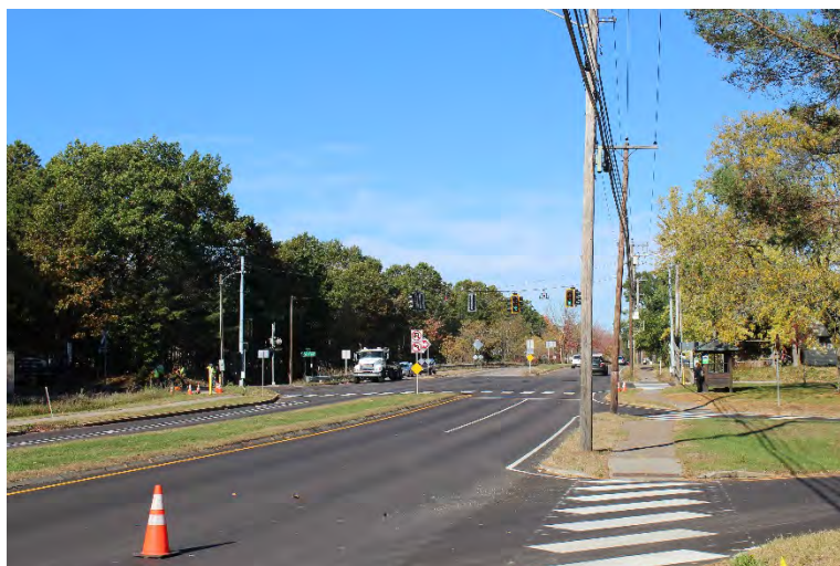
Figure 8 Westerly Perspective of VT Route 15 / West Street Extension Intersection
