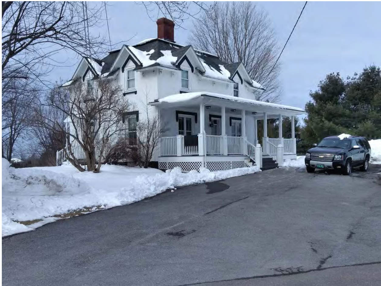
Figure 10. Structure 5, looking west.
