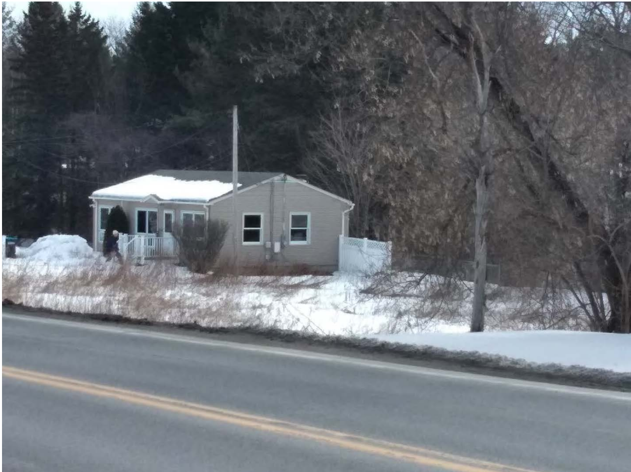
Figure 15. Structure 8, looking east.
