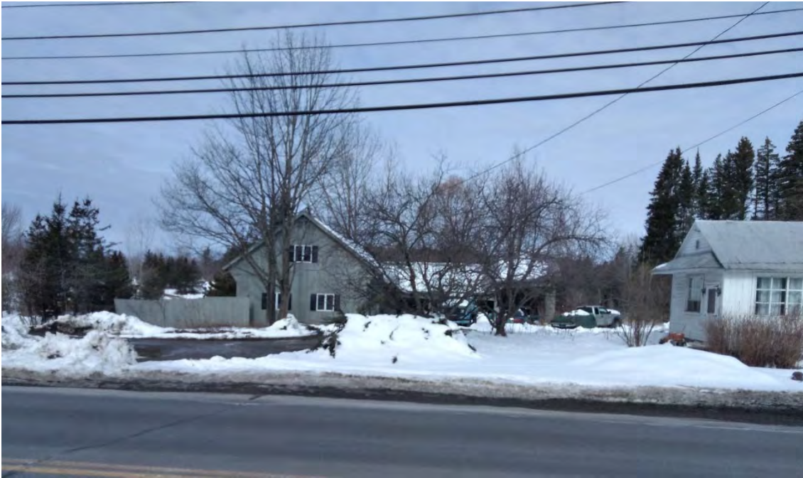
Figure 7. Structure 3, looking northwest at the converted barn complex.
