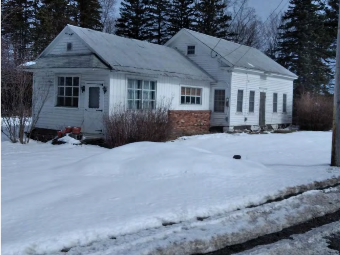
Figure 6. Structure 3, looking north.
