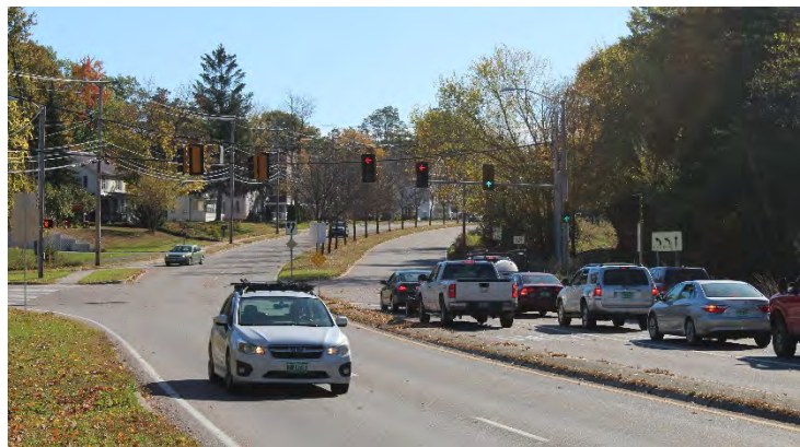
Figure 7 Easterly Perspective of VT Route 15 (Pearl Street) / Susie Wilson Road Intersection
