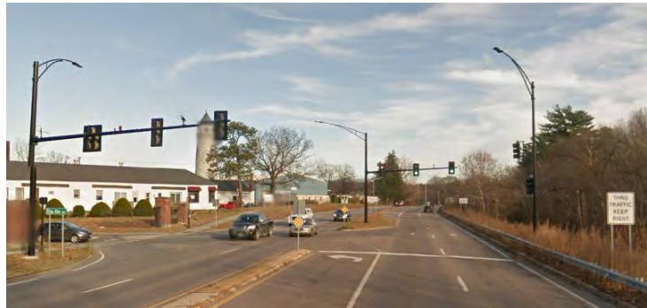
Figure 6 Westerly Perspective of VT Route 15/ Ethan Allen Avenue Intersection (Google Street View, 2015)
