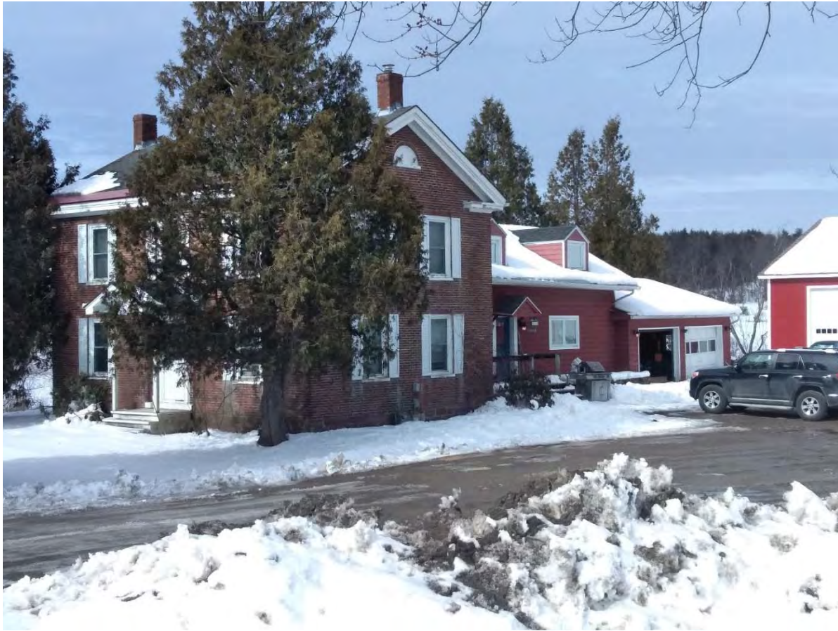
Figure 9. Structure 4, looking west. A closer view of the house.
