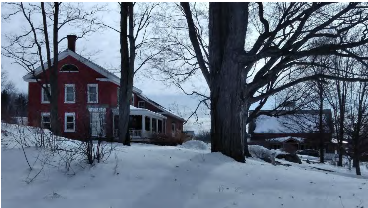
Figure 16. Structure 9, looking east-southeast.
