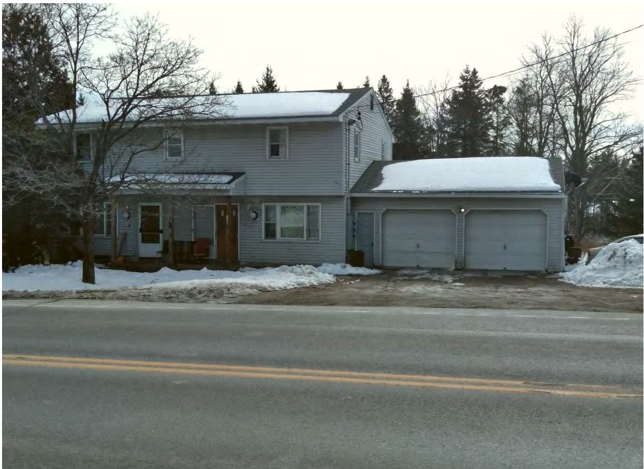
Figure 14. Structure 7, looking east.
