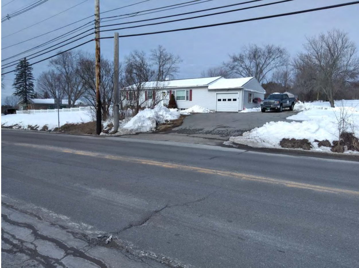
Figure 4. Structure 2, looking west.
