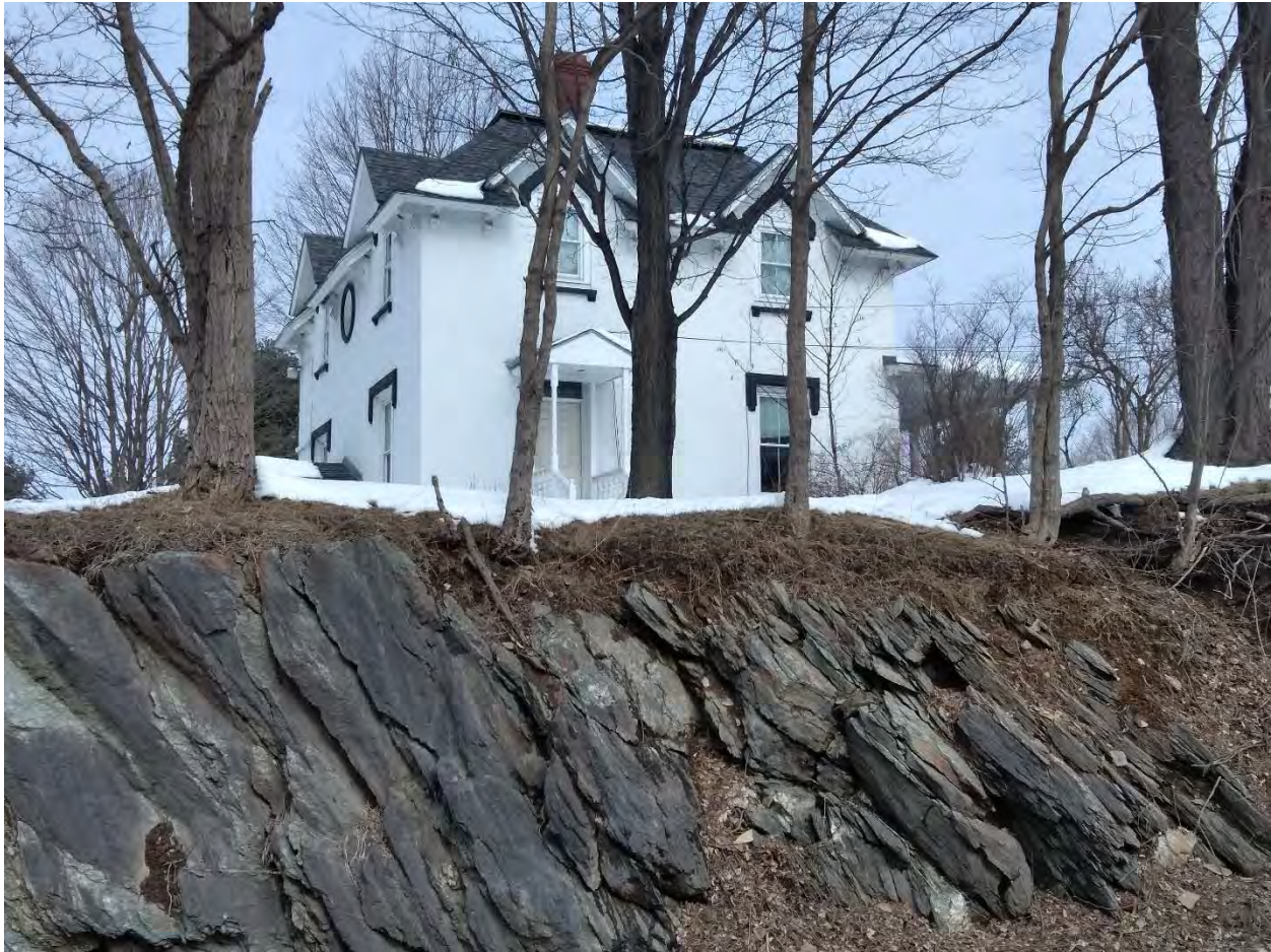
Figure 11. Structure 5, looking north. The west elevation with circular window is visible in this view.
