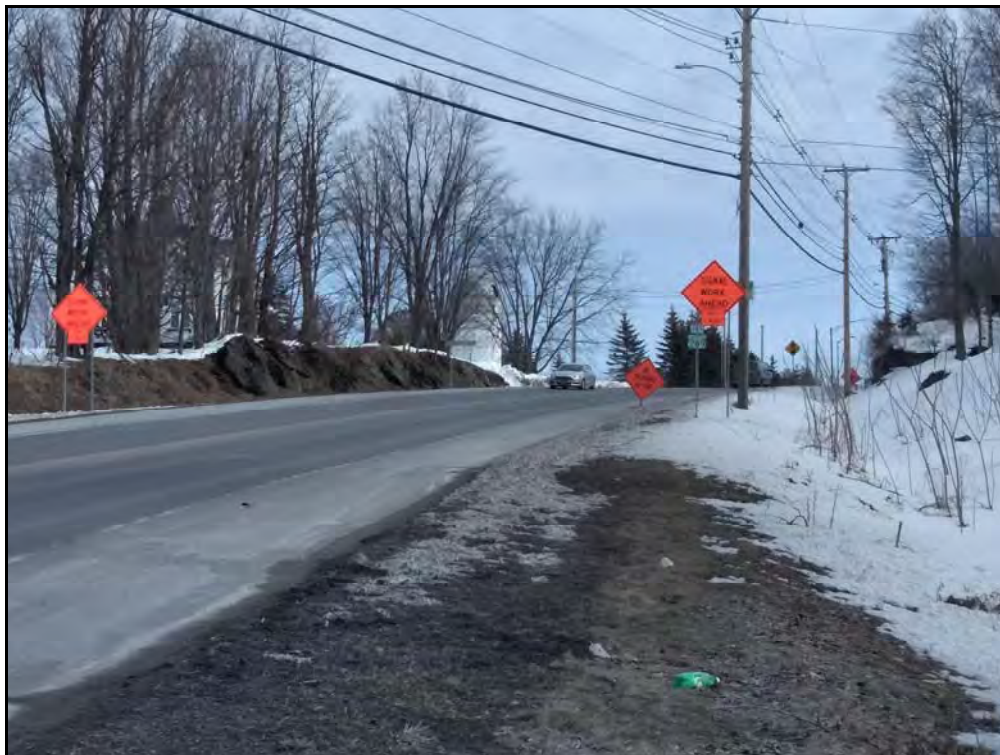
Photo 6. Photo shows a large shallow roadside gully on the east (right) side of the road, and large bedrock outcrops on the west (left) side of the road. View is to the north.
