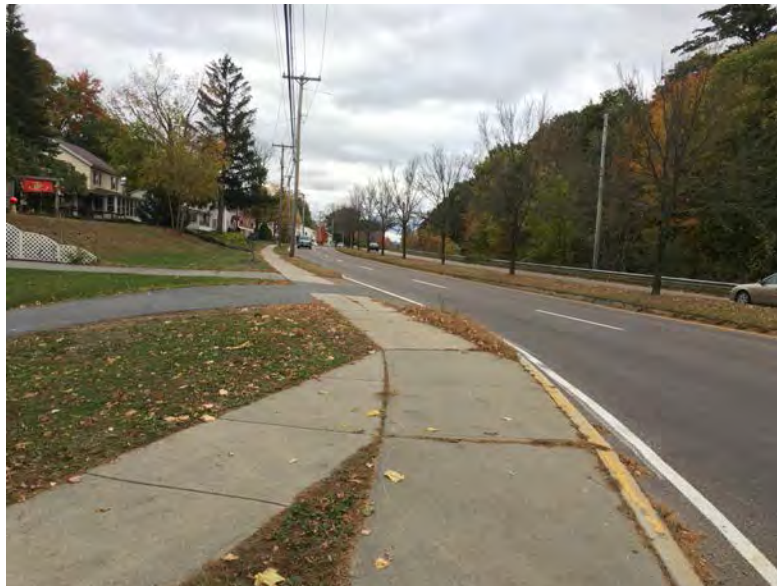
Photo 2. View looking east along the north side of VT 15 showing existing sidewalk and residences (to left). 10/18/17
