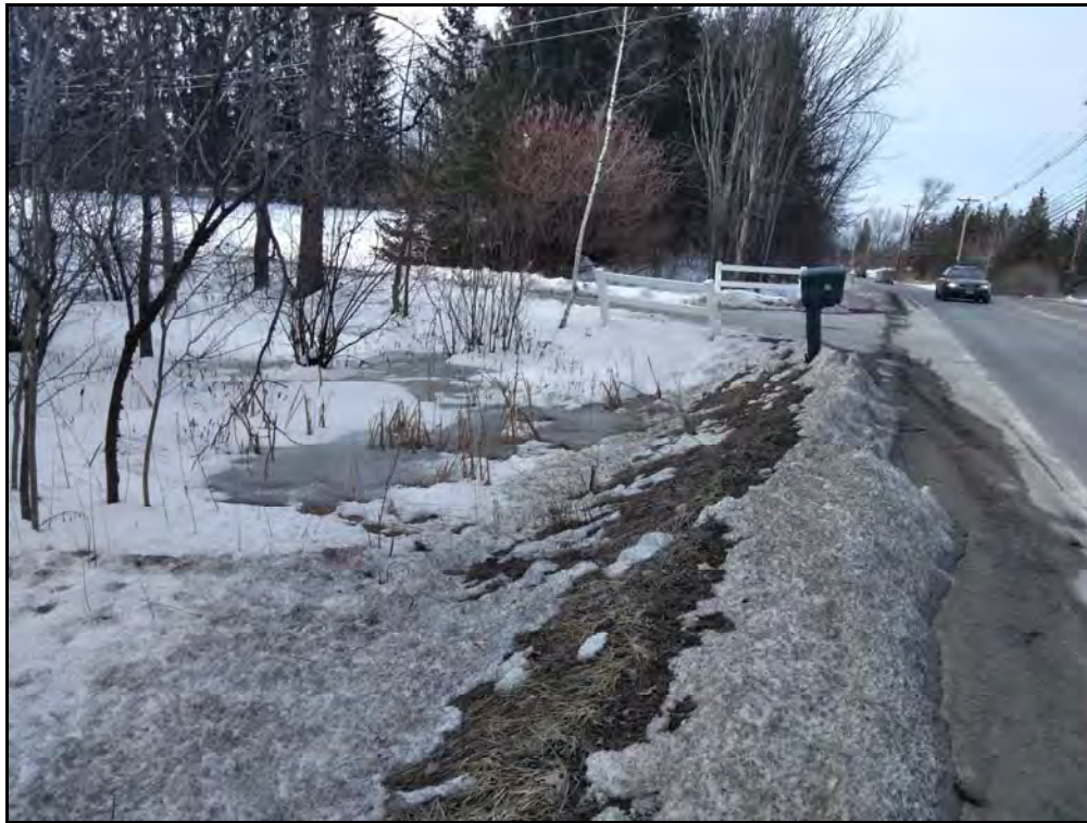
Photo 5. Photo shows a large roadside gully. A large portion of the project area contained similar drainage gullies adjacent to the roadway. View is to the south.
