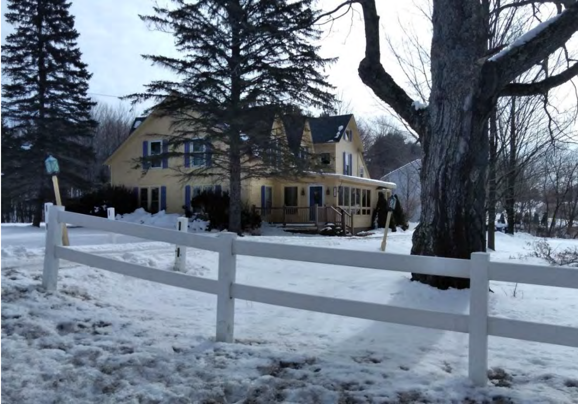
Figure 12. Structure 6, looking east.
