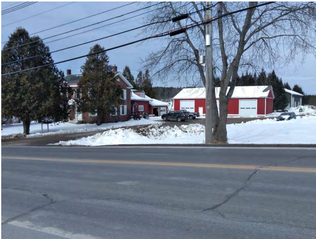
Figure 8. Structure 4, looking west.
