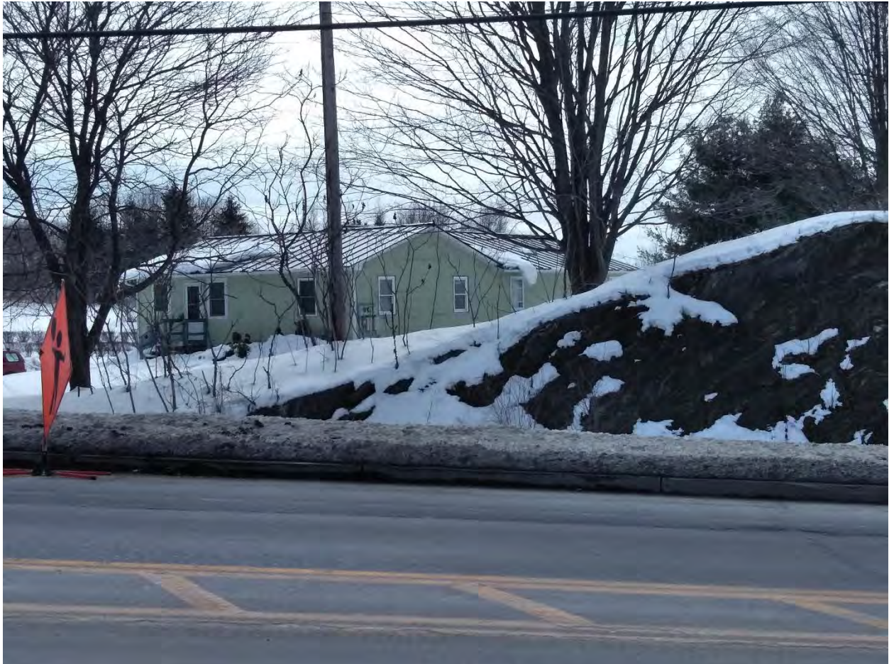
Figure 19. Structure 10, looking east-southeast.
