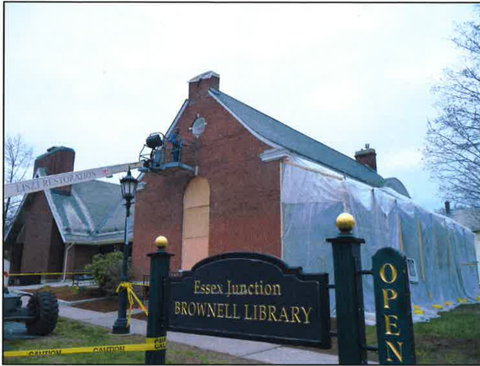
Brownell Library Exterior Rehabilitation
