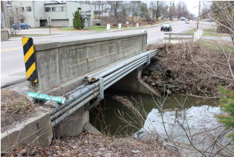
Illustration 2: Indian Brook flowing east under Main Street as seen from the northwest.
