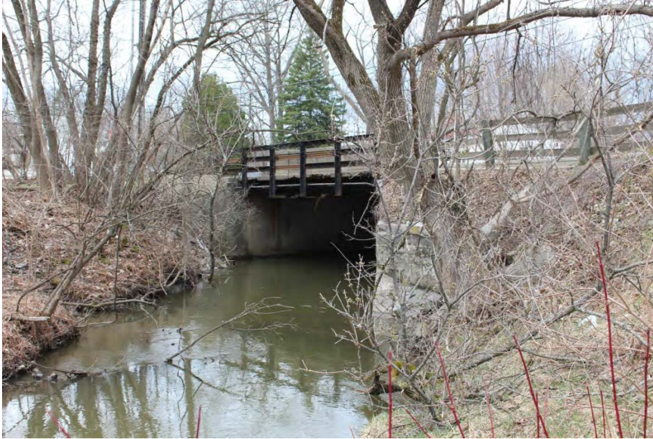
Illustration 1: Indian Brook flowing west under Main Street as seen from the northeast
