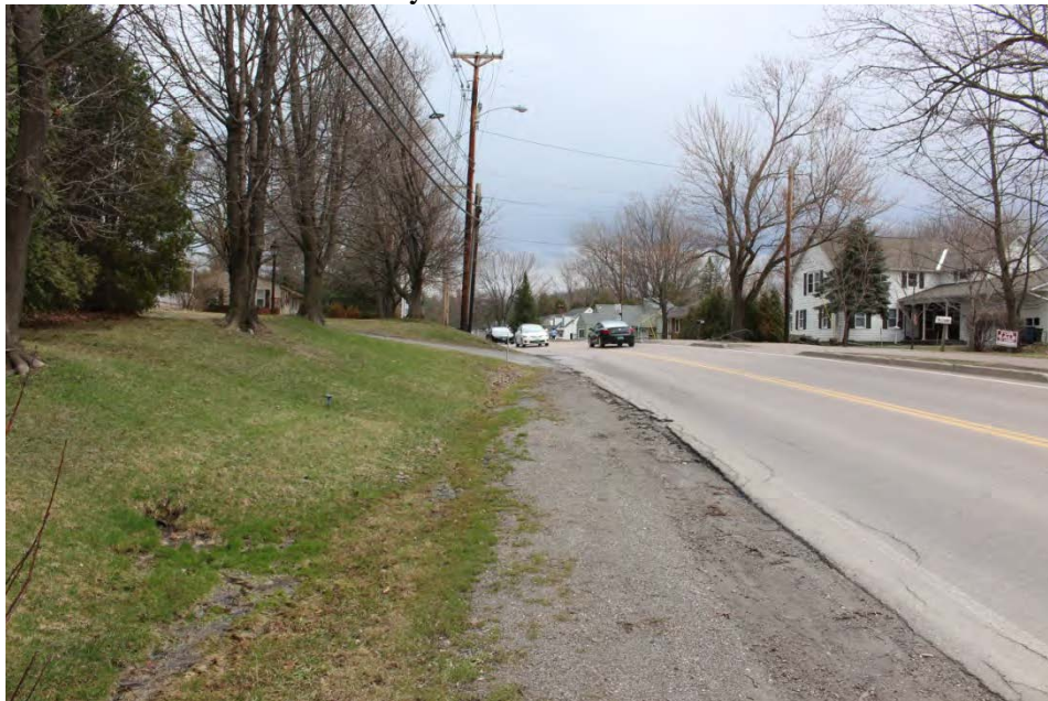
Illustration 5: View of Utility Pole To Be Relocated at 140 Main Street
