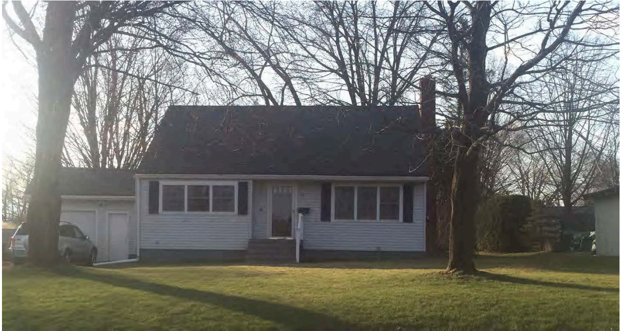
Figure 4. Typical of the mid-century Main Street neighborhood, this c.1958 dwelling at 92 Main Street displays features of a simple Cape with eaves-front roof, centered entrance, and attached garage. Courtesy Heritage Landscapes. (R-EJ Sidewalk-92 Main Street-21April2015)
