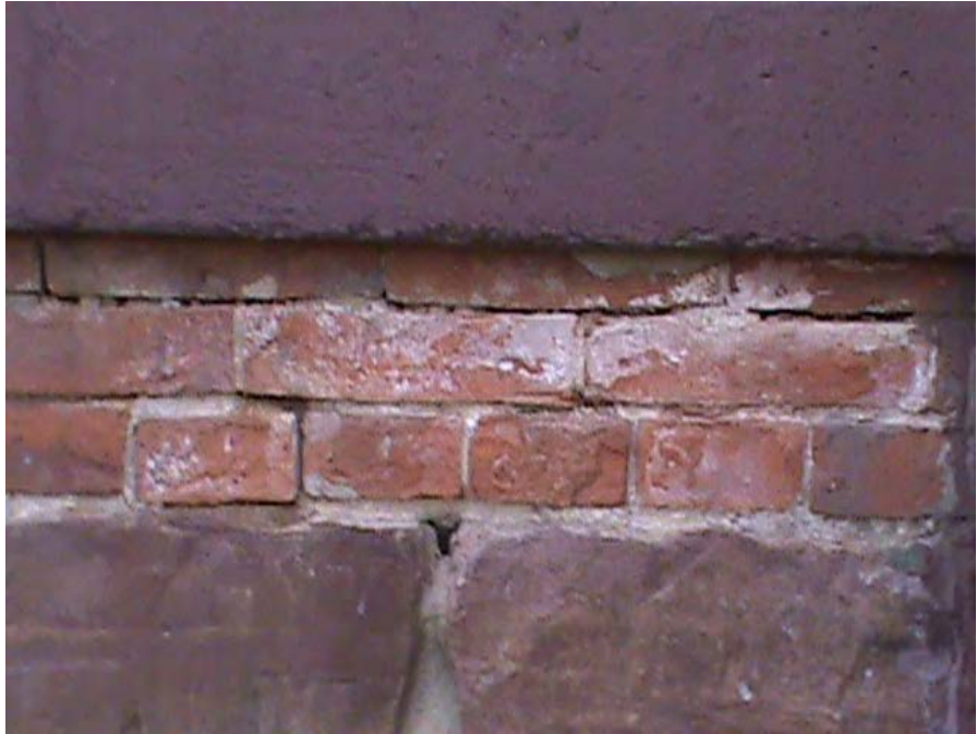
b) Spalled brick to the left of entry steps, ~ 10 c.t.
