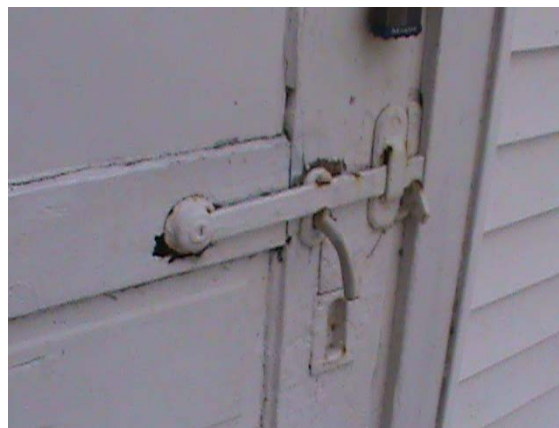
a) Severely rotten by the door handle.
