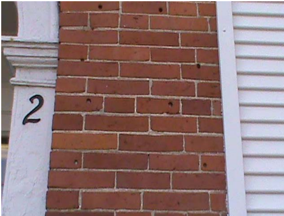
c) Several brick have holes, ~ 9 c.t.
