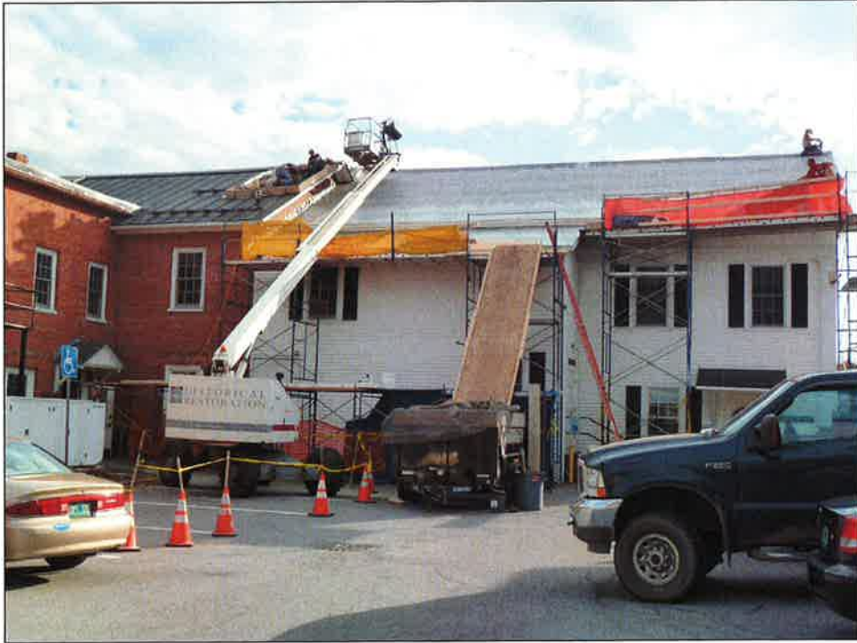
Lincoln Hall Restoration Work
