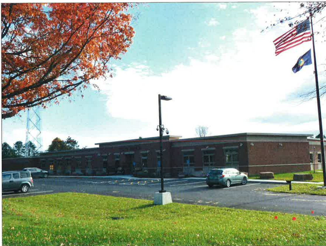
The New Essex Police Facility
