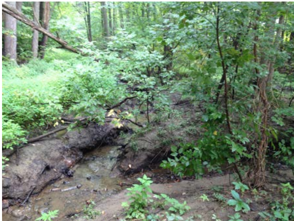
Figure 1 - Wooded area at culvert inlet (looking north)
