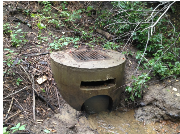
Figure 2 - Shawn's Way culvert inlet
