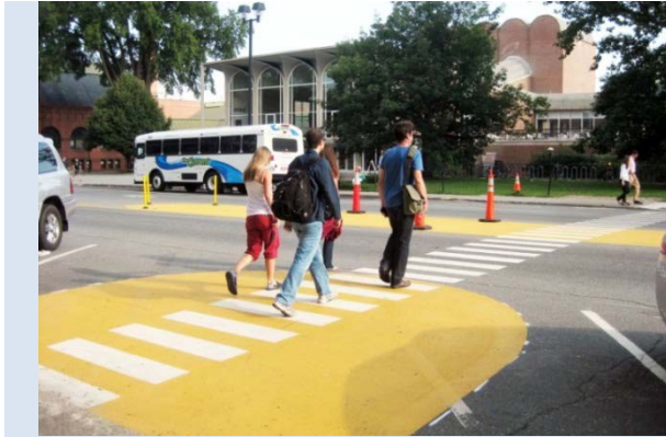
Temporary Bulb-out in Hanover, NH
