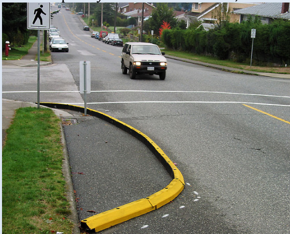
Temporary Curb Extension
