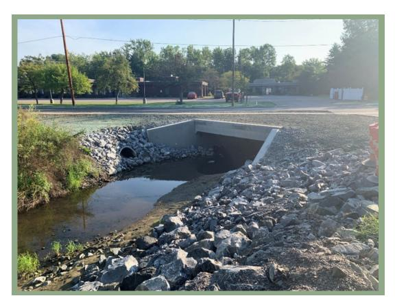
The culvert Indian Brook passes through on Densmore Drive near Main Street was destroyed in a Fall 2019 storm. FEMA provided 75% of the funds to replace the culvert with a properly sized culvert pictured above. There was associated water, sewer and stormwater line replacement work done as part of the project. The project was completed in summer 2021.
