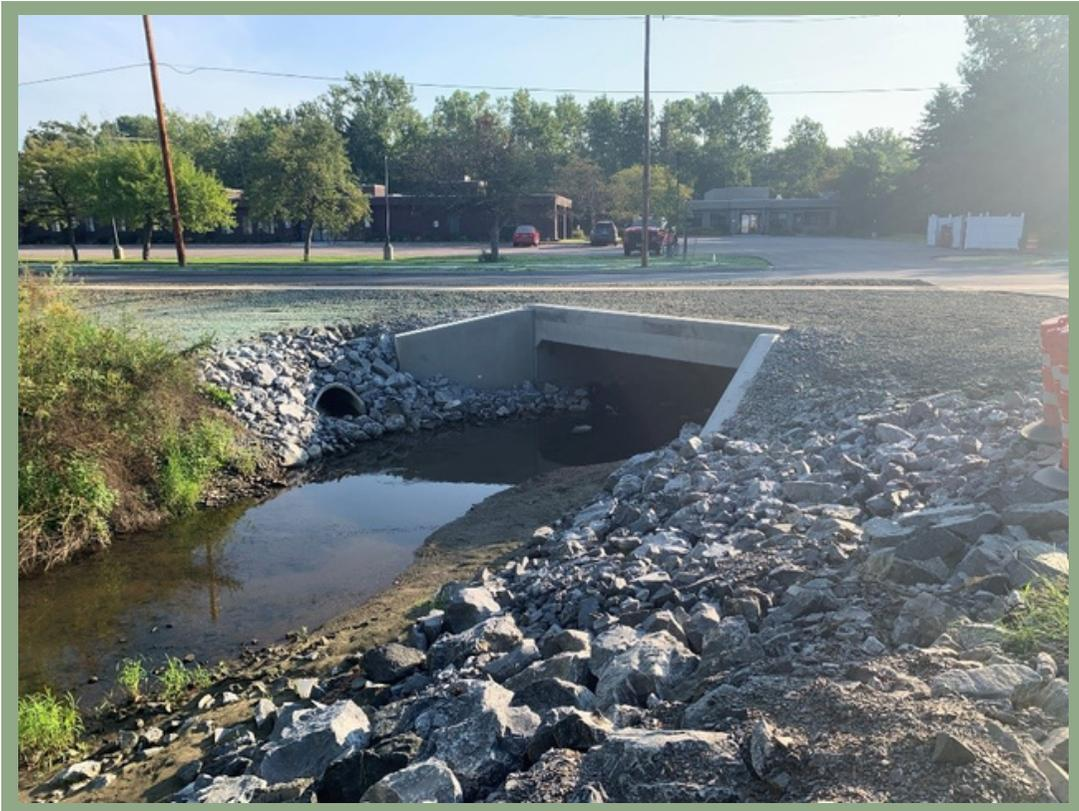
*The culvert Indian Brook passes through on Densmore Drive near Main Street was destroyed in a Fall 2019 storm. FEMA provided 75% of the funds to replace the culvert with a properly sized culvert pictured above. There was associated water, sewer and stormwater line replacement work done as part of the project. The project was completed in summer 2021.*
