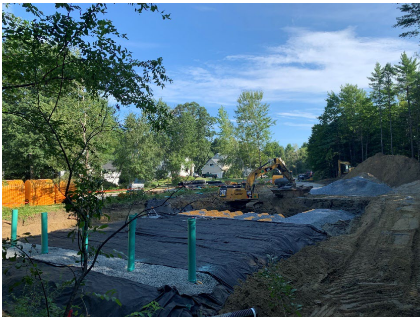
Figure 6: Sydney Drive Pond Retrofit during construction in August 2020.
