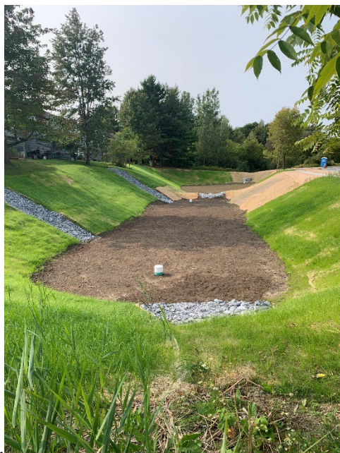
Figure 10: Mansfield Brickyard Gravel Wetland after install Sept. 2020
