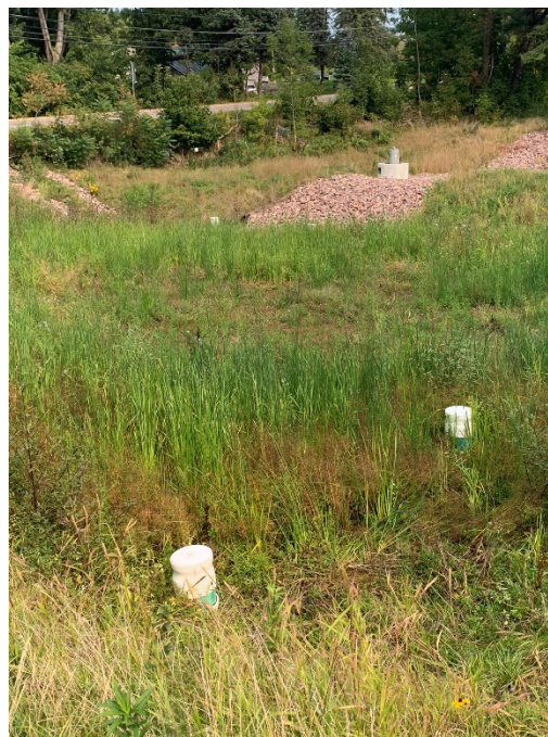
Figure 9: Fairview Dr. Gravel Wetland one year after install -Summer 2021
