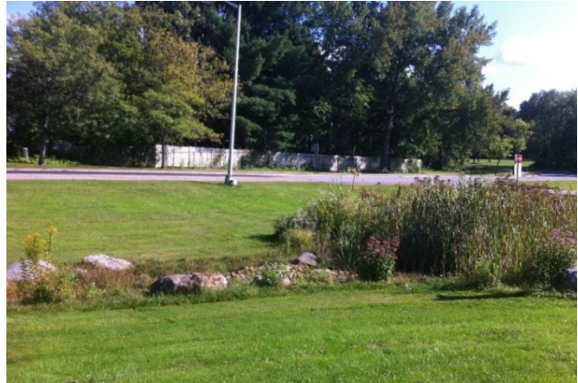
Figure 11: Essex High School Rain Garden
